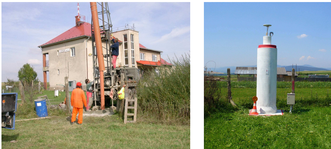
Fig.3 Permanent station Lie1 (Liesek) – realization and final status
